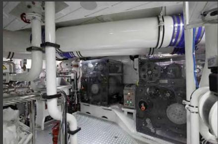
Sybaris is equipped with two 120 kW variable speed generators – a first on a Perini Navi yacht – supplying electrical power via a DC bus to the vessel's main electrical grid with the potential to store excess power in lithium polymer batteries.
